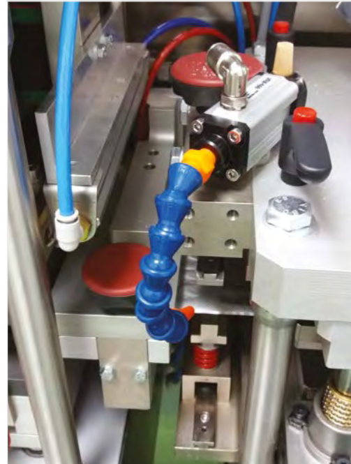
Cooling of blisters
