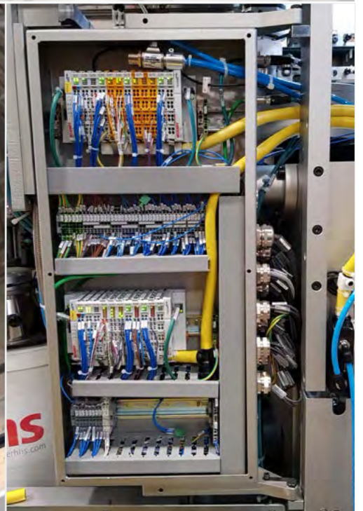
Cooling of control cabinets
