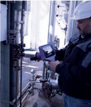
STEAM TRAP INSPECTION
